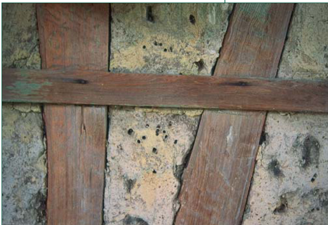
The Hypolite Bordelon House in Marksville (top) is an example of Creole architecture in the late 1700s and early 1800s. The walls (above, left) are bousillage, a mixture of mud and deer hair or Spanish moss. The dining room in the house (right) was one of the two main rooms. The netting in the bedroom, the other main room (opposite page), protected the sleeping occupants from mosquitoes.
